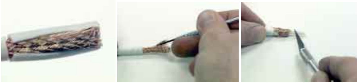
Figure 7a - 7c. Prepare the coax and install the F-connector.
