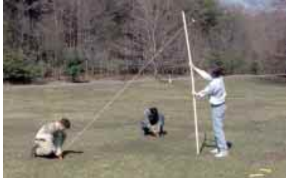
Figure 10a and 10b. Lay out each dipole on the ground. Set up one pole at a time.
