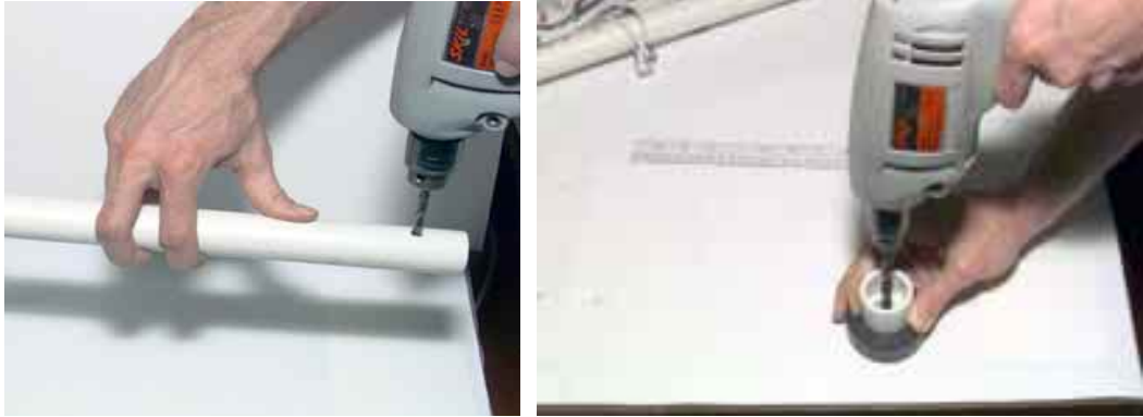
Figure 8a and 8b. Drill the PVC piping and end cap.
